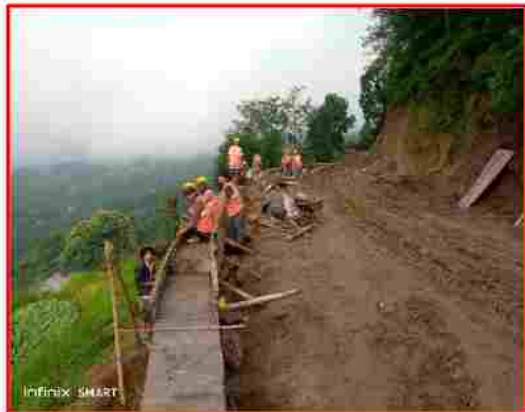
Construction of Plum wall at CH 2+460-CH 2+500
