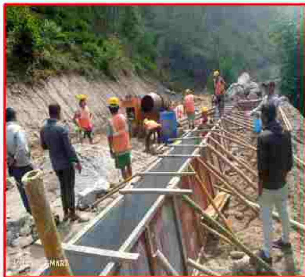
Visited of Ward Chairman, Ward No.1,2 At Site
