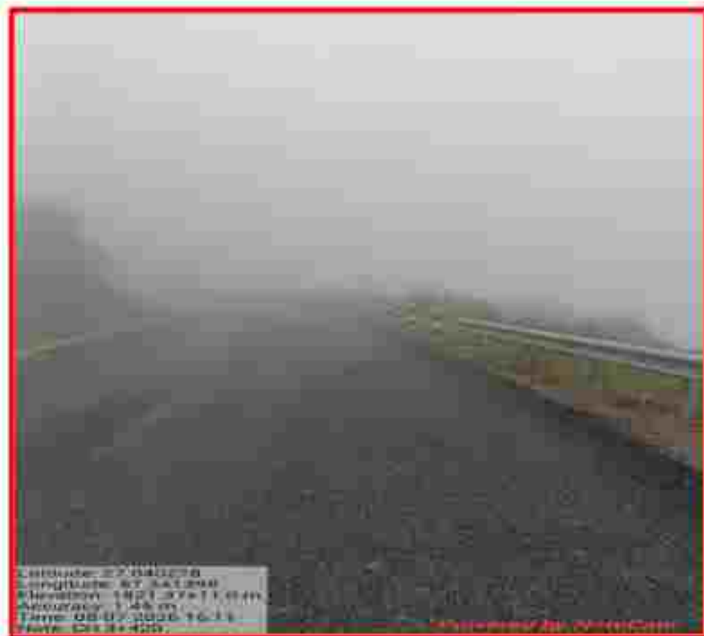
Asphalt Construction Work
