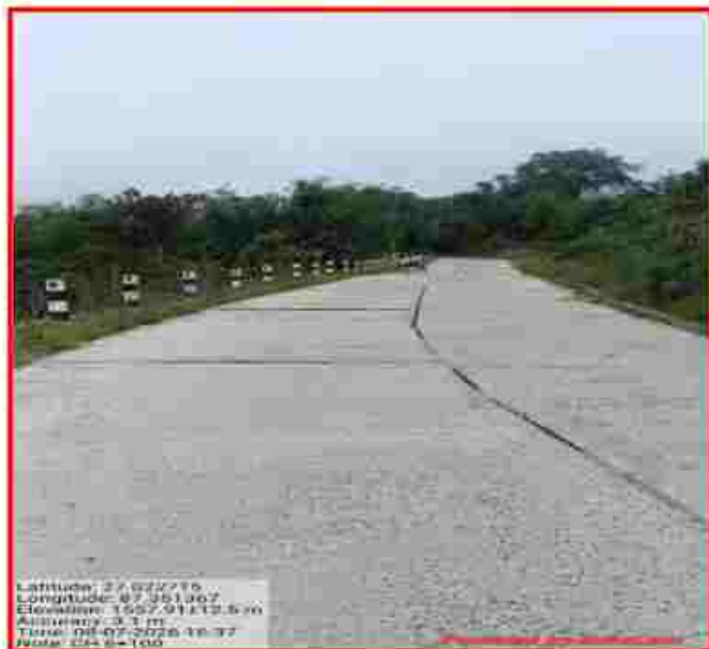
20CM Thick M25 RCC Rigid Pavement
